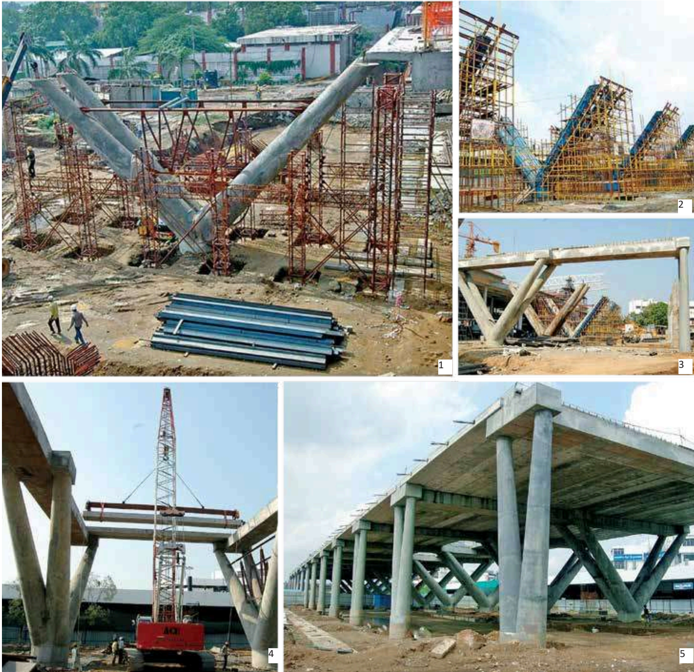
CONSTRUCTION SEQUENCE OF V-COLUMNS
