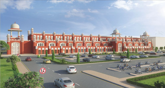
The second entry station at Plot-2
