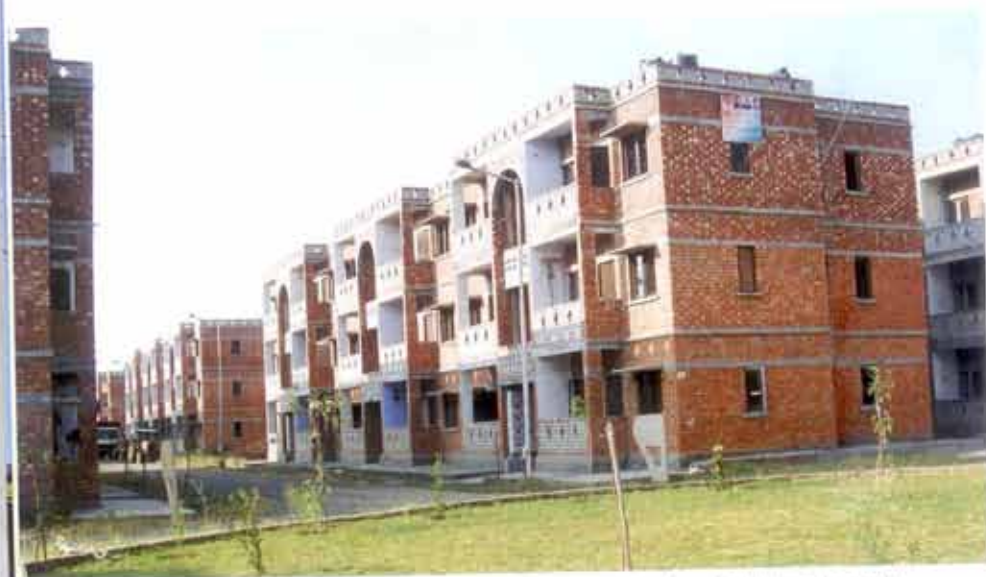
Affordable Housing at Omicron, Greater Noida, by Adlakha Associates headed by Promod Adlakha.
